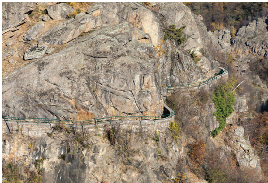
Fig. 124 and 125: The water supply canal carved into the canyon's cliffs
